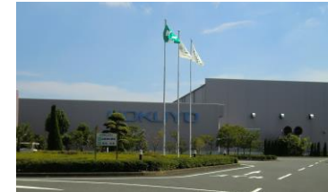
Shibayama Plant Exterior view of the plant
